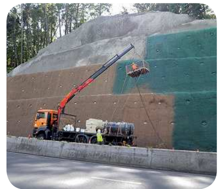
Hydroseeding application (Euro-Tec, France)
